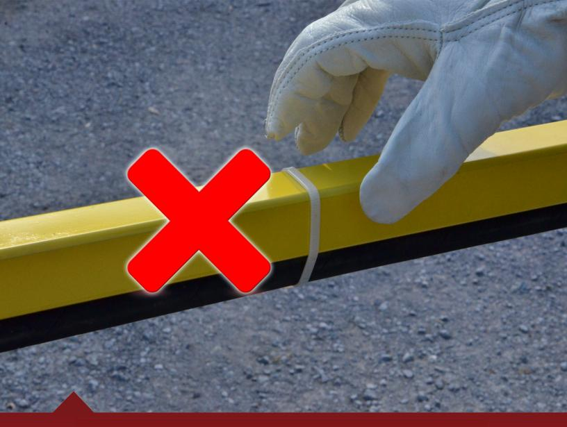
Never attach hydraulic hoses to hand rails. This changes the grip dimension of a hand rail which is hazardous. Should a breach occur, this exposes the hand to an energy hazard including a slip hazard.
