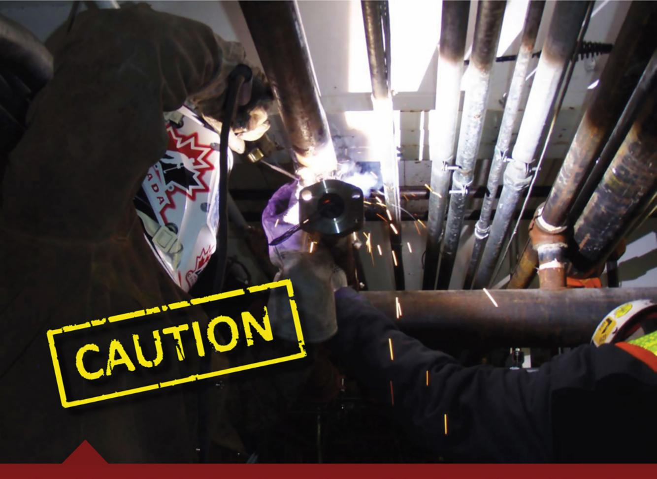
Accidental electrode arcing of hydraulic tubing is extremely dangerous. The resulting arc can easily blow holes in the thin walled tubing. Under pressure, these holes will produce the atomized spray of hydraulic fluid which could then cause: fire, inhalation, burns, and slip hazards.
