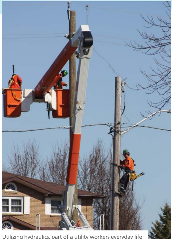
Utilizing hydraulics, part of a utility workers everyday life
